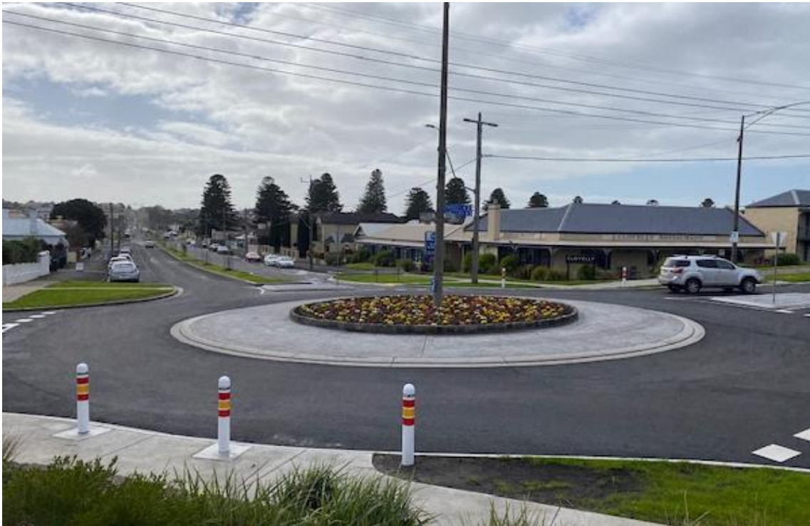
Photo 5: Roundabout upgrade – intersection of Banyan Street and Merri Street
