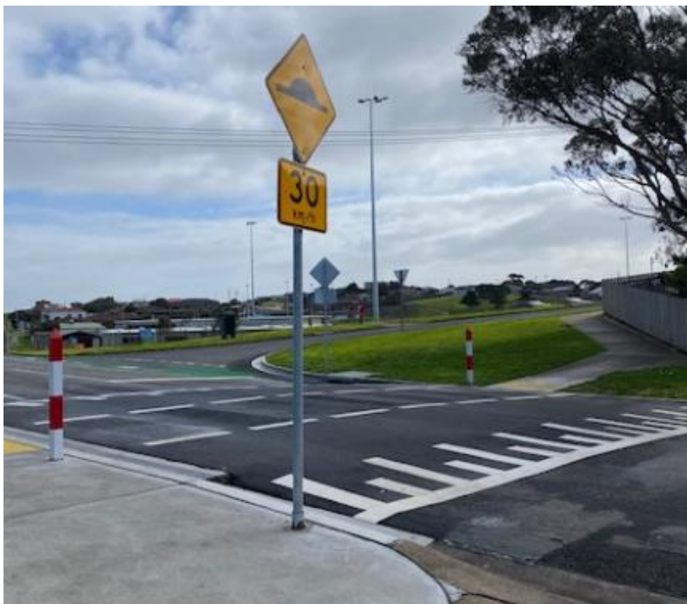
Photo 2: Raised school crossing – Merrivale Drive near Merrivale Primary School
