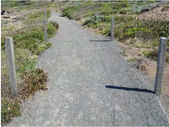
Photo 5: Pathway surfaced with basalt gravel, foreign geological material
