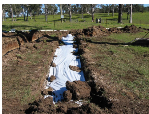
Figures 19 & 20: Latter stages of installation of soil absorption trenches (Source: Civicon 2019); soil mound effluent disposal (SCA 2019).
