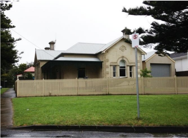
Substantial c1880s+ corner villa, with stucco finish to walls, steep corrugated galvanised iron roof, projecting gable fronts, return curved verandah and decorative quoins and feature windows. Villa stands as a key feature of precinct
