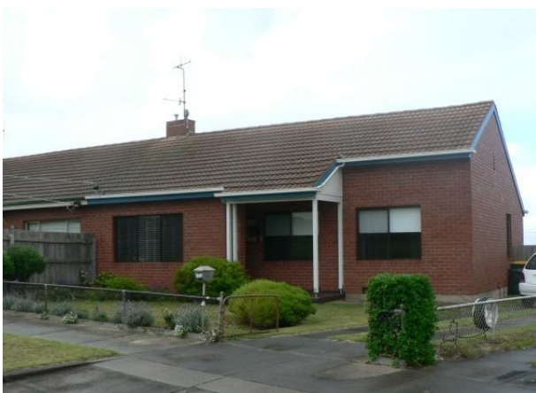
Note – timber windows replaced with aluminium frames
