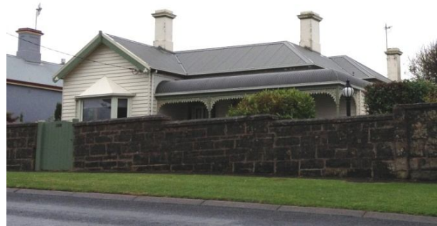
Note masonry fence to front, timber weatherboard cladding to dwelling and masonry chimneys - late 19 th century villa typical to precinct
