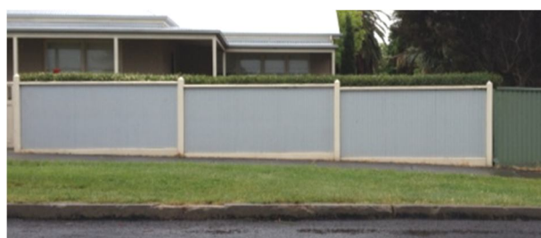
Low corrugated, galvanised steel sheet panels framed in timber posts/ rails compatible with era of the precinct
