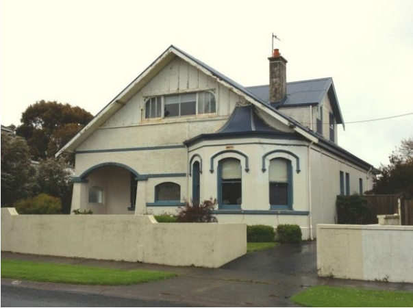
Early 20 th century dwelling – note steep roof with rooms in attic, decorative bay window and front verandah. Front fence also integral in design and material
