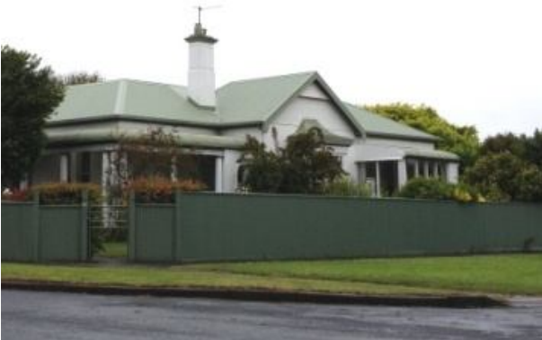
C 1880-1910 villa, with return bull nose verandah and projecting bay window centred on gable. Note chimneys and use of corrugated roofing – green colour not typical to precinct - commonly galvanised, or painted red late 19 th Century.
