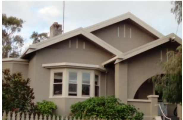
Typical bungalow front – note multi-gable roof and integration of verandah under main roof.
