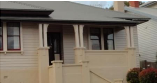
Verandah common to period – note masonry base, 1/2 posts and simple timber brackets
