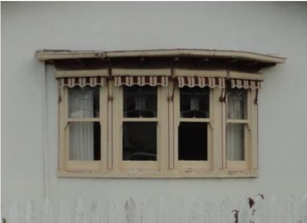
Typical bow window to front facade of bungalow
