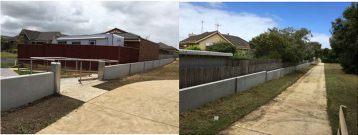
Figure 3. Constructed flood walls. (Source; Water Technology 2017).
