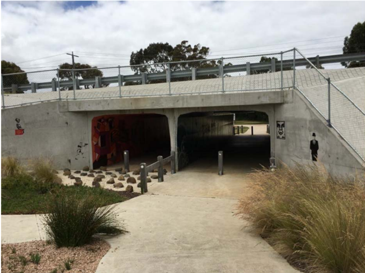
Figure 4. Constructed culverts under Mortlake Road. (Source; Water Technology 2017).
