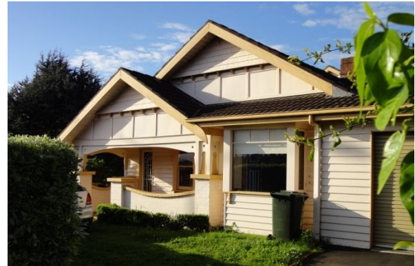
Interwar bungalow dwelling – note decorative gables with timber battens and shingle facing, timber brackets to verandah and projecting bay window – all contributory features within the precinct
