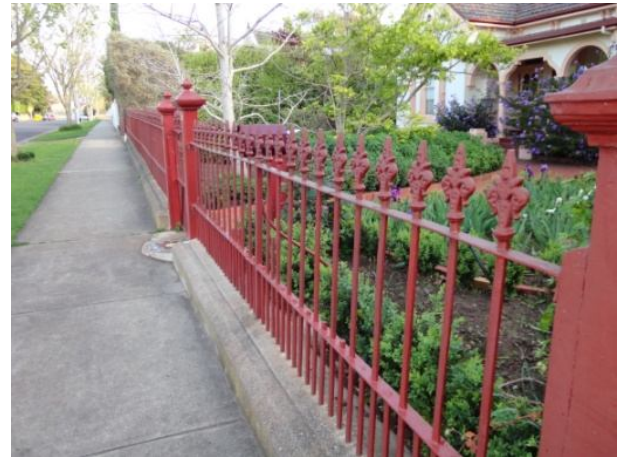
Cast iron/ wrought iron fencing found in the precinct – associated with substantial 1880s era dwellings only
