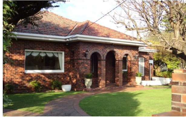
Interwar era cottage of high architectural quality – but with features common to earlier dwellings in the precinct – pitched roof, decorative arches, projecting front verandah
