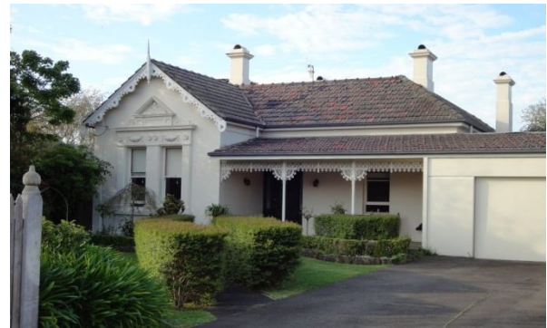
C1880s villa - set in generous grounds – note the steeply pitched roof, dominant chimneys, front verandah and vertically proportioned windows. Integration of garage not ideal, as alters the scale of the front facade and verandah.
