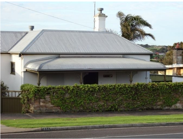
C1880s symmetrical villa with hipped CGI roof and bullnose verandah – part of the precinct character
