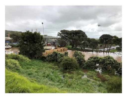
Figure 1-12 Photo of flooding temporary levee at the Midfield Meats Rendering Plant with helicopter dropping sandbag
