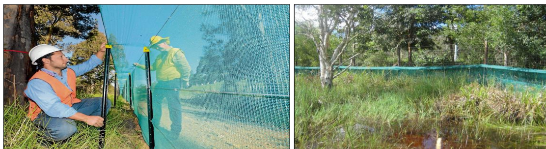
FIGURES 39 & 40 – Barrier fencing used to direct or restrict frog passage within urban development construction site. 44
