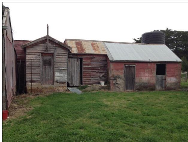
Plate 17: View of 78 Boiling Down Road, Warrnambool facing south - sandstone barn and associated wooden & corrugated tin extension.
