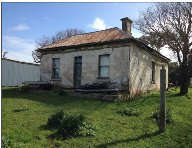
Plate 12: View of 174 Aberline Road, Warrnambool facing north – primary sandstone structure.
