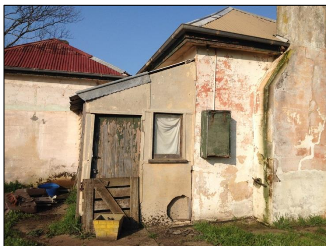
Plate 15: View of 174 Aberline Road, Warrnambool facing south-west - primary sandstone structure with extension.
