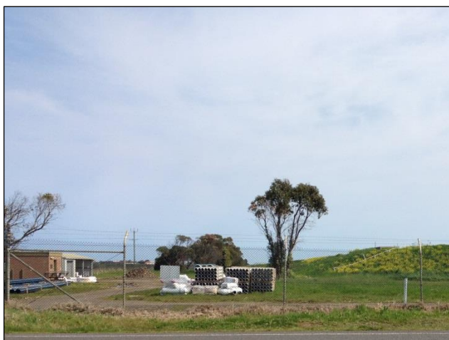
Plate 3: Study area facing west showing poor GSV of undulating plains landform at Wannon Water storage facility and SGD.
