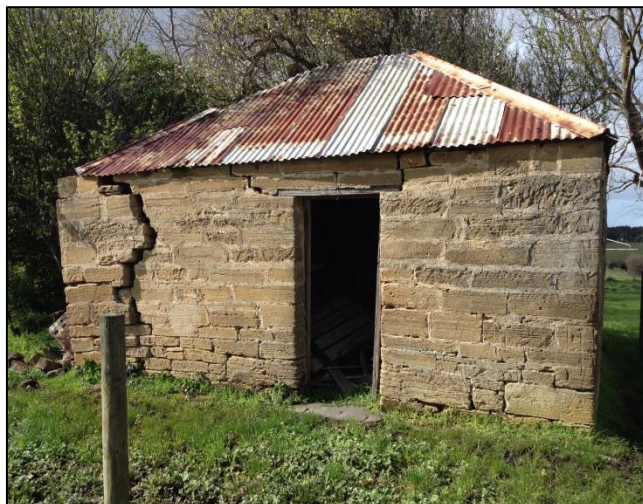
Plate 13: View of 174 Aberline Road, Warrnambool facing south-east – secondary sandstone structure.
