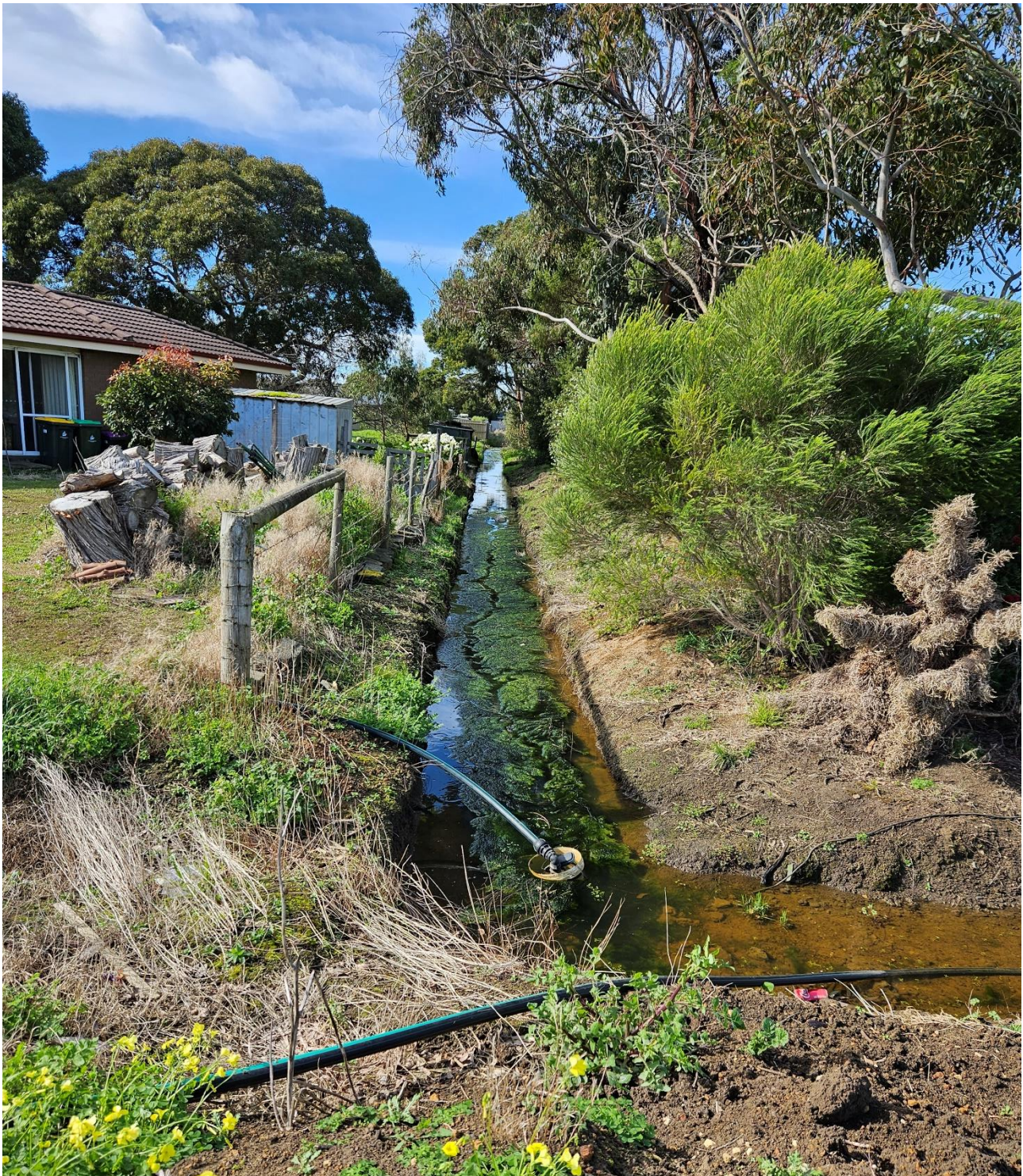
Figure 3-6 Easement drain at relatively new dwellings on Elizabeth Street with pump in drain
