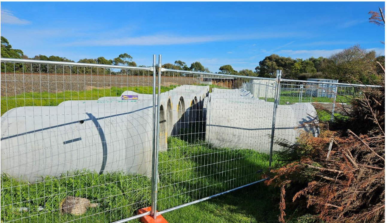
Figure 3-3 New 1200mm RCP pipe sections awaiting installation to replace aging outfall to Hopkins
