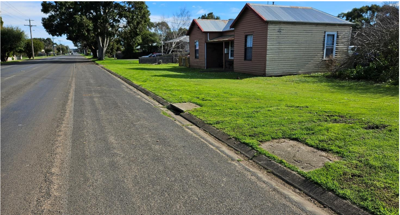
Figure 3-5 Taken at the front of 122 Ziegler Parade, showing extremely flat grade of Ziegler Pde – a known flooding hotspot
