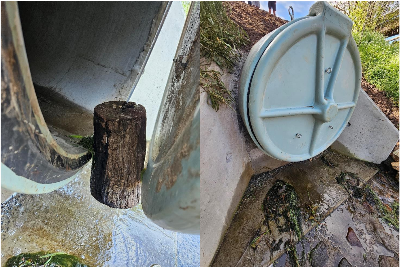
Figure 3-7 Floodgate on end of new Tooram Rd North Outfall – left side shows block of wood used to wedge the gate open permanently
