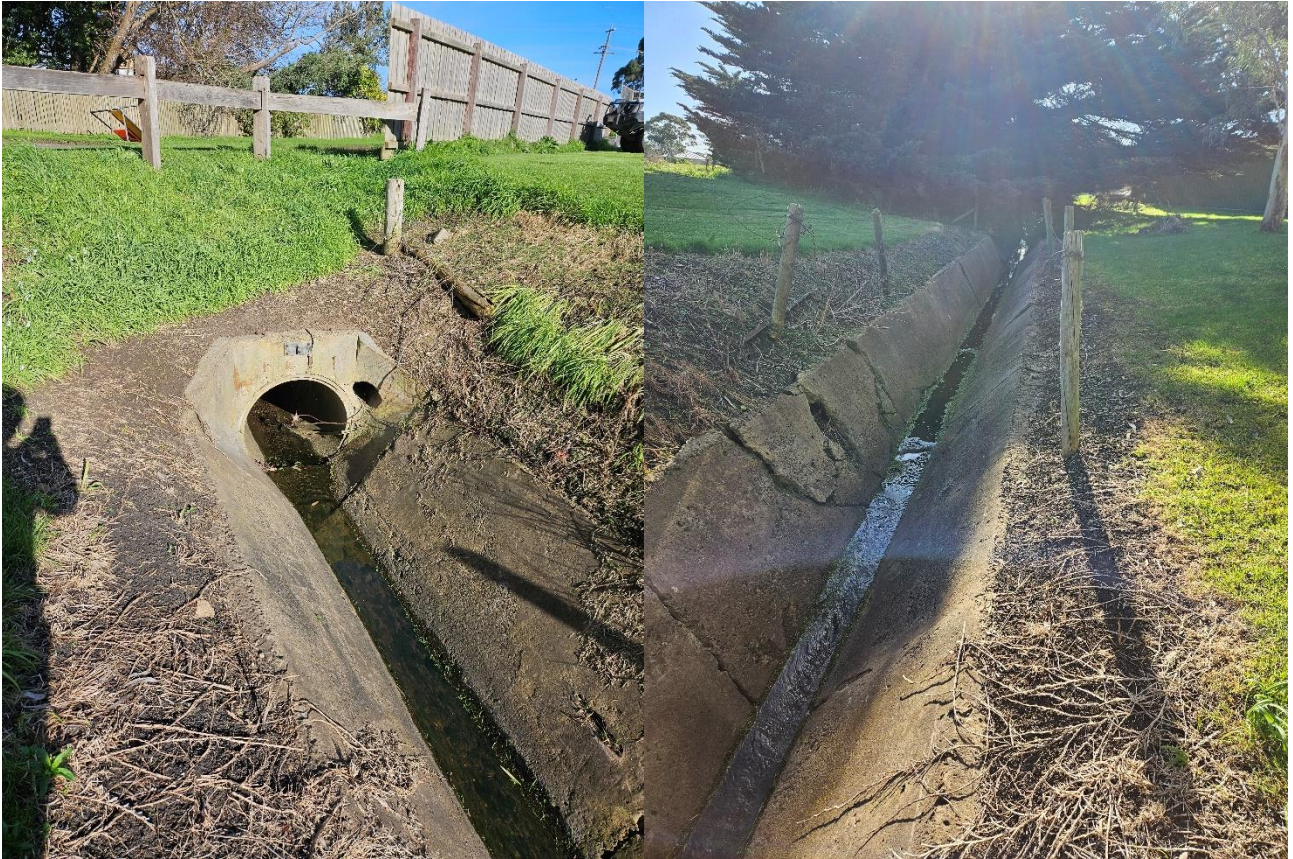
Figure 3-2 Main Open Drain in Allansford and 825mm RCP draining the majority of the town
