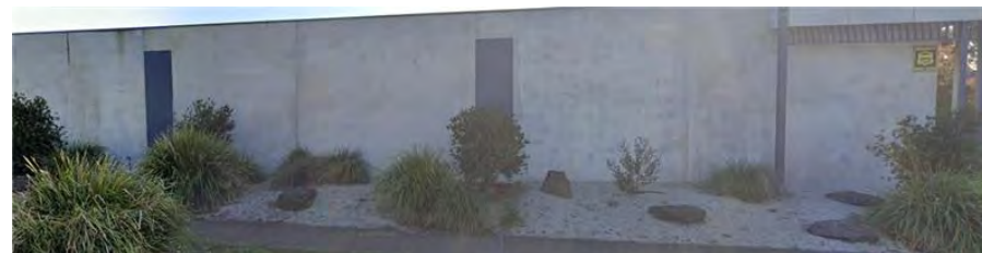
Buildings should avoid large blank expanses of wall, where it faces a street.
