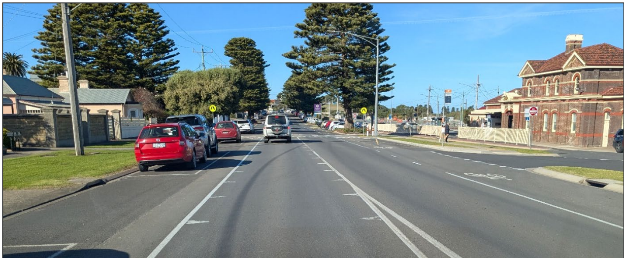
Figure 2.2 Merri Street (facing southeast at site frontage)
