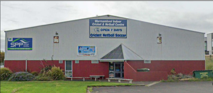
PHOTO 02 - ENTRY / FACADE FACING MORTLAKE ROAD
