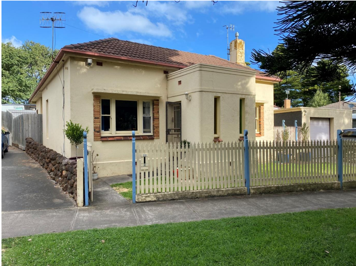
Current Site Streetscape.
