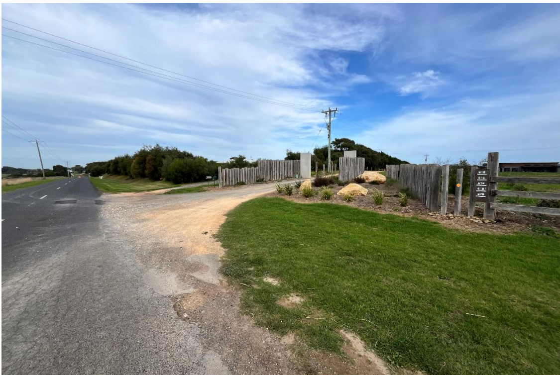
Image 2: View of existing access to 610, 612, 1/616, 2/616, 618 & 620 Hopkins Point Road (looking south-east).
