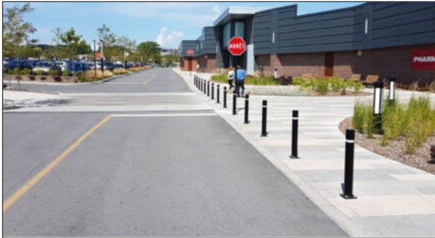
Figure 6.1 Example of Parking Aisle to Footpath Barriers
