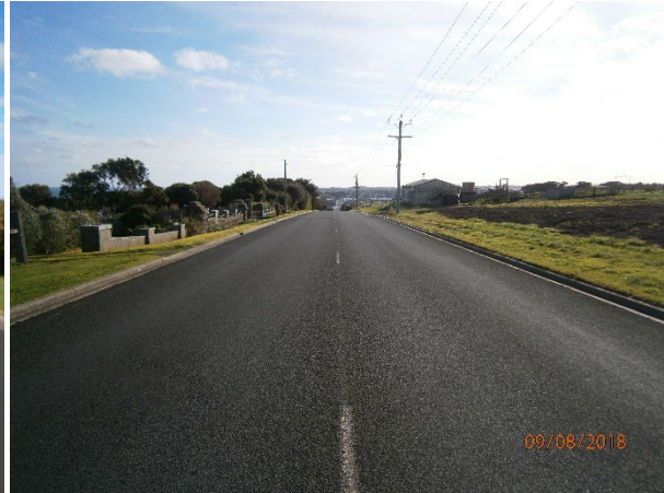
Figure 4: Hopkins Point Road - View West from near Eastern Site Boundary
