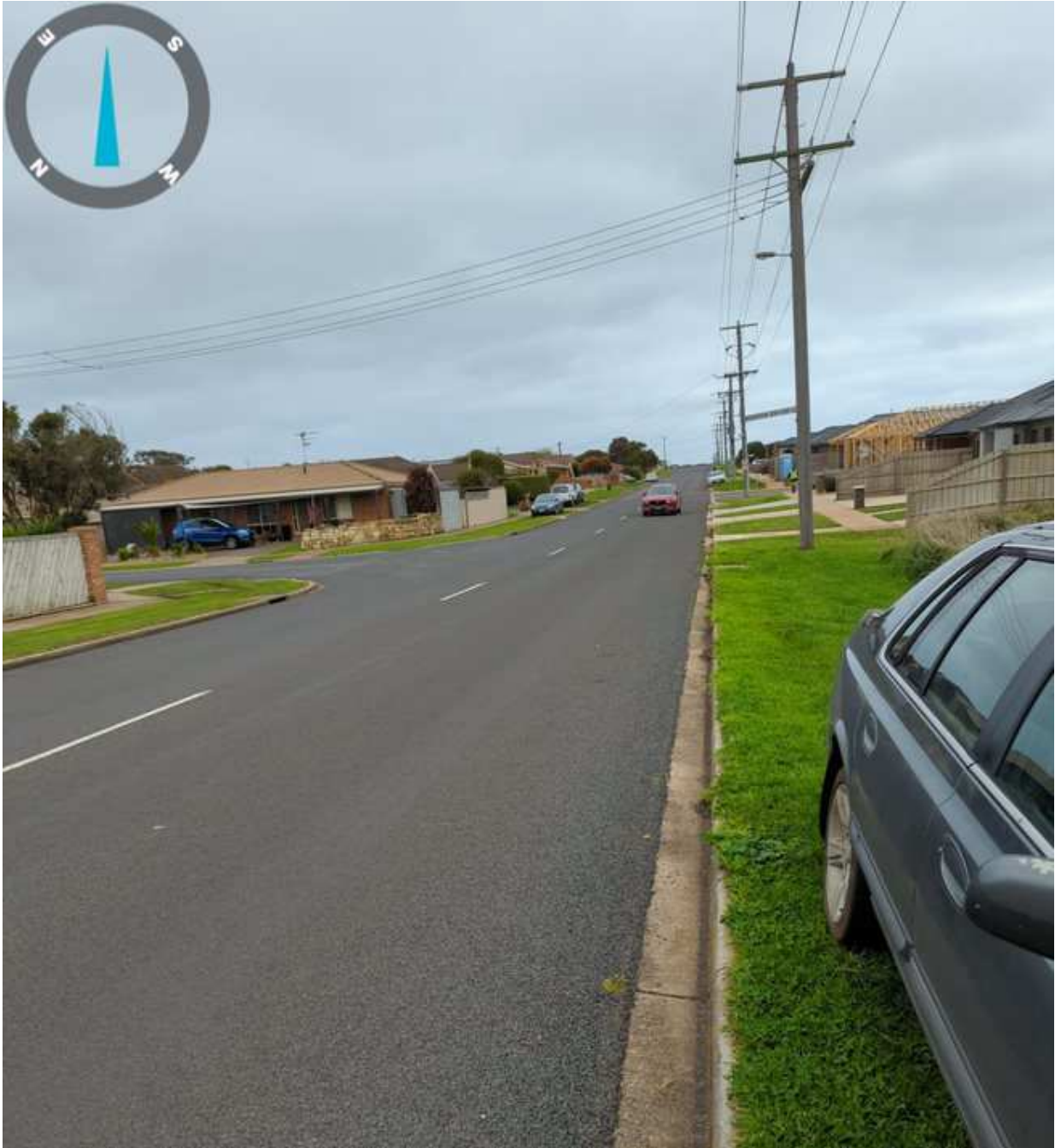
PHOTO 2: MORRISS ROAD (LOOKING SOUTH) – PROPOSED COMMON PROPERTY INTERSECTION LOCATION Morriss Road has a 9.5m sealed width and a 20.12m road reserve width between B-Type kerbs, making it a mix between an Access Street and a Collector Street Level 1.
