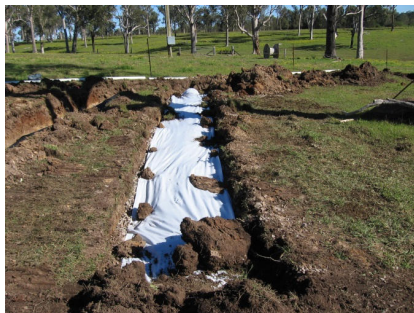
Figures 19 & 20: Latter stages of installation of soil absorption trenches (Source: Civcon 2019); soil mound effluent disposal (SCA 2019).
