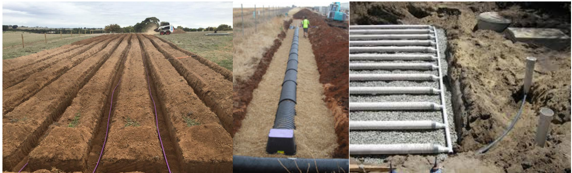
Figures 16-18: ETA beds can be used with septic tanks to reduce and concentrate affluent disposal area; another useful upgrade option for small lots and aging systems (Source: Hydroscape 2019, William Cromer 2019, Mornington Peninsula Shire Council 2015).
