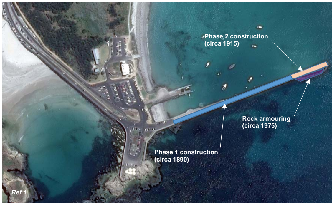
Figure 4 Location of Warrnambool Breakwater
