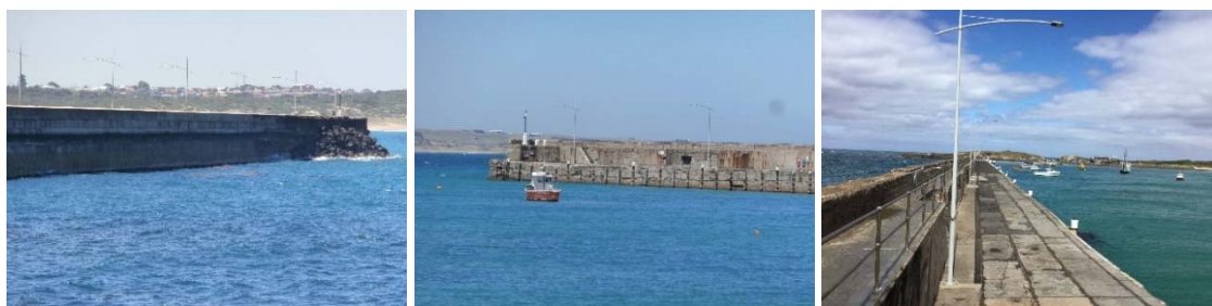
Figure 5 Warrnambool Breakwater - Current Configuration (2018)
