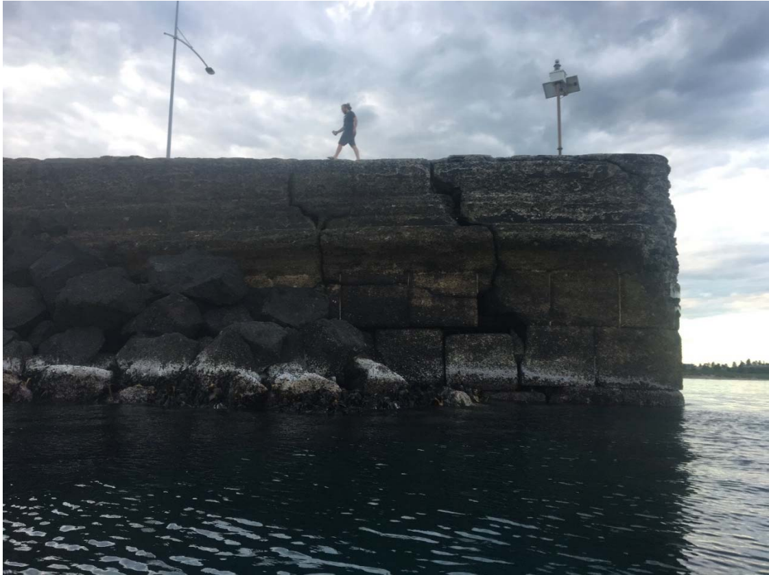
Figure 11 Armour Rocks at Breakwater Head
