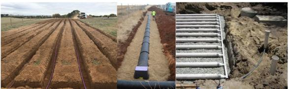
Figures 16-18: ETA beds can be used with septic tanks to reduce and concentrate affluent disposal area; another useful upgrade option for small lots and aging systems (Source: Hydroscape 2019, William Cromer 2019, Mornington Peninsula Shire Council 2015).
