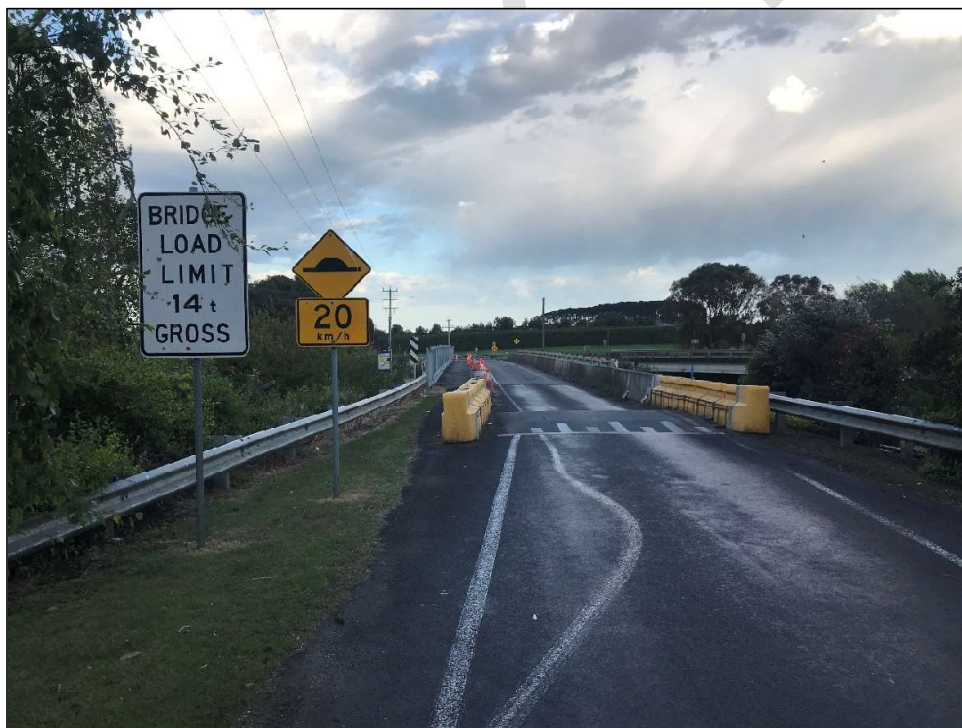
Figure 6: Deck view (note posted load limit and speed restriction)
