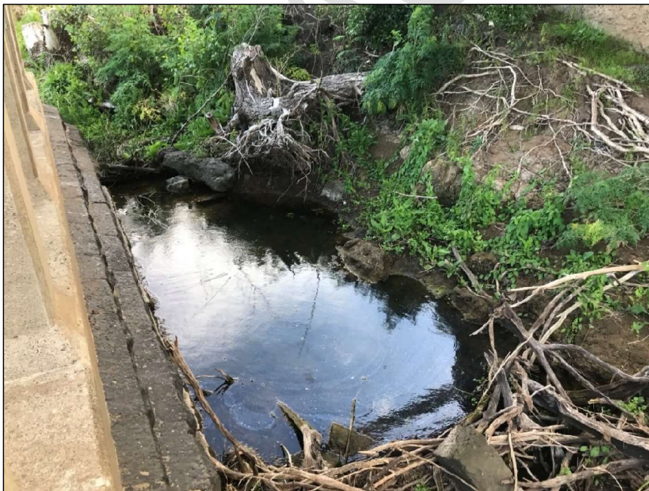
Figure 26: Scour at base of batter slope in front of Abutment 1
