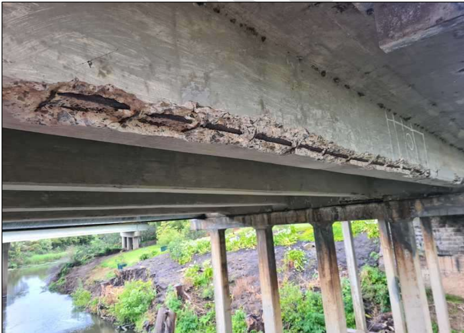
Figure 22: Tee-beam soffit spalling with exposed and corroding reinforcement
