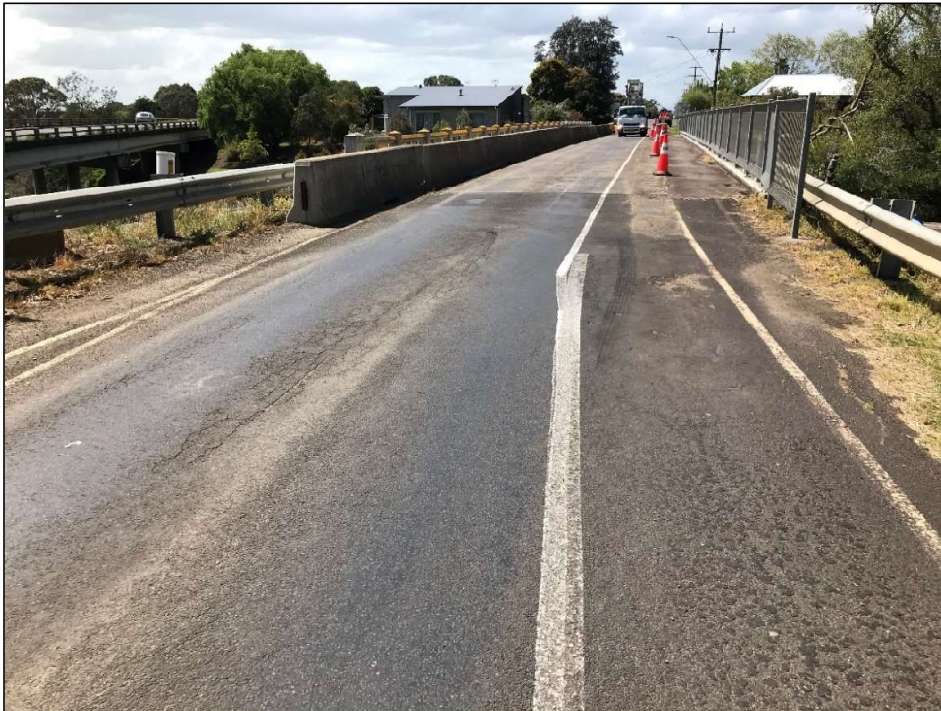
Figure 20: Road surface defects on bridge approach / departure
