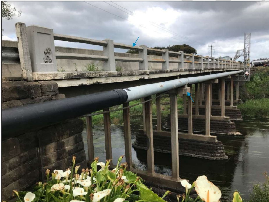
Figure 17: Note original barriers and pier crosshead extensions supporting service pipe
