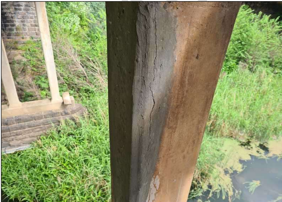
Figure 24: Cracking of 2013 column patch repair
