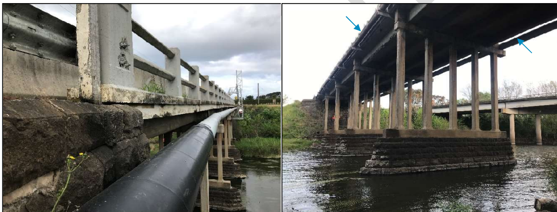
Figure 6: Services attached to the bridge
