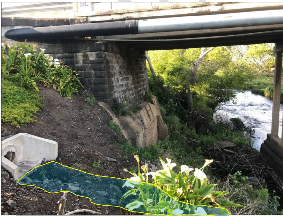
Figure 19: Erosion evident at drainage outlet
