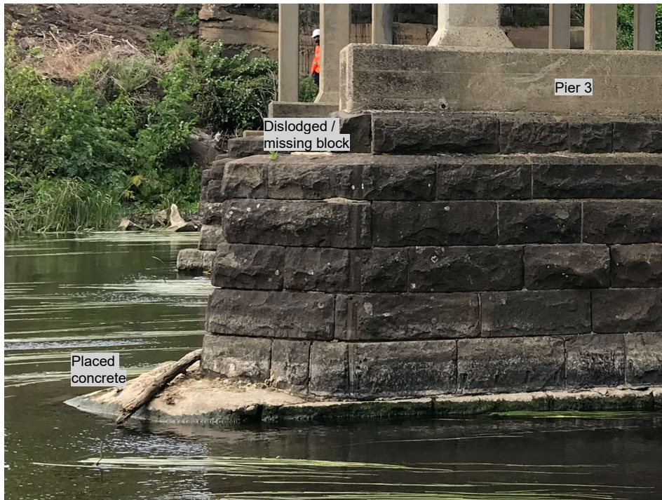
Figure 25: Loss of mortar between masonry units
