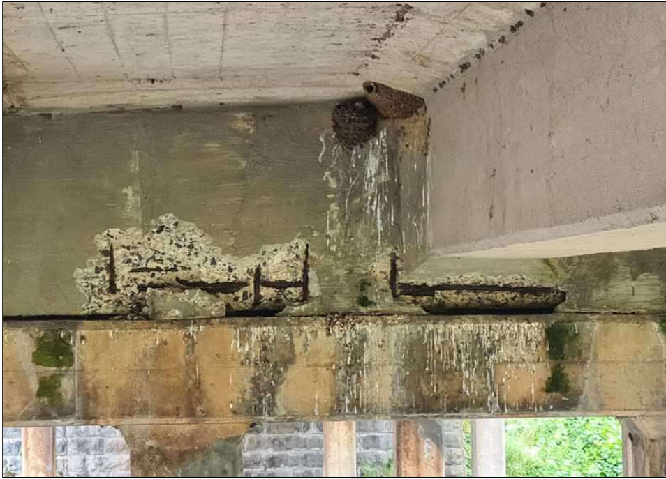
Figure 23: Diaphragm spalling with exposed and corroding reinforcement
