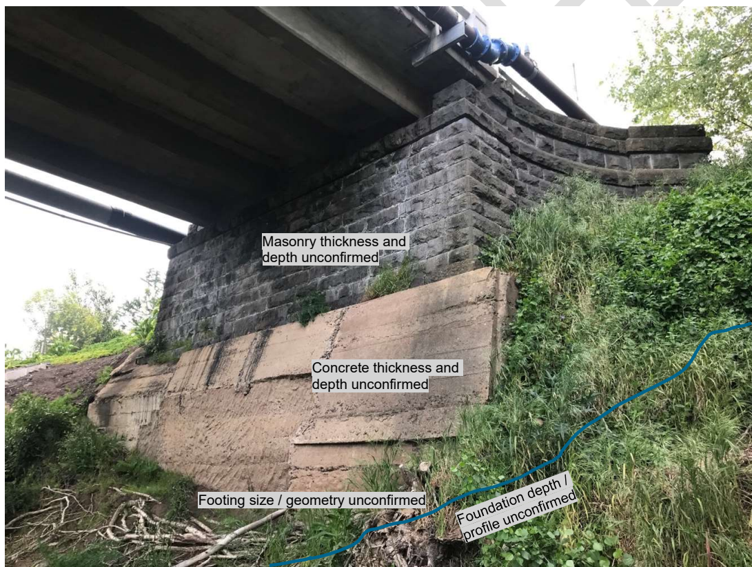
Figure 27: Abutment details unconfirmed
