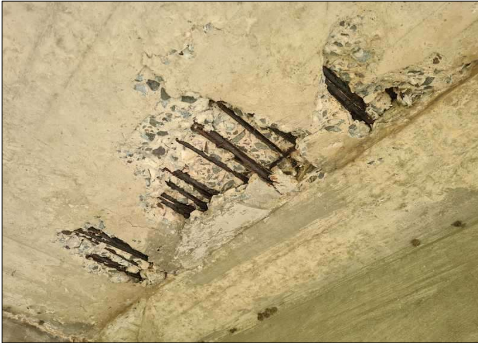
Figure 21: Deck soffit spalling with exposed and corroding reinforcement
