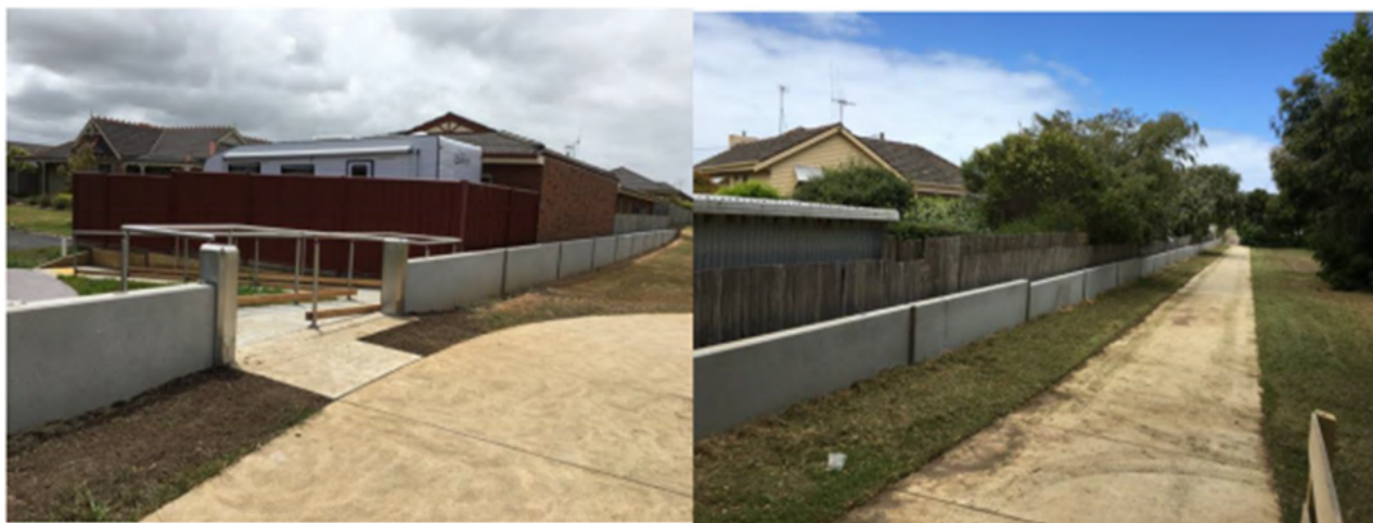
Figure 3. Constructed flood walls. (Source; Water Technology 2017).
