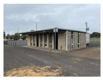
Photo 4: Store building (former bar) viewed from north west showing masonry external walls and a flat pitched roof.
