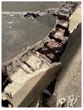
**Photo 3:** View on broken section of platform at midspan showing Bondek completely corroded through leading to brittle failure of concrete.
