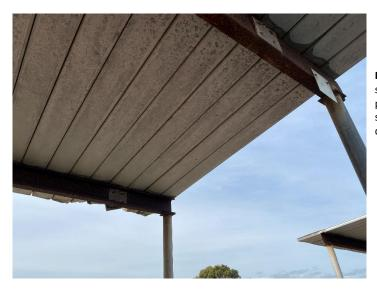
**Photo 6:** View of typical roof structure showing corroded support purlins and roof sheeting in single span arrangement over excessive distance for capability of sheeting.
