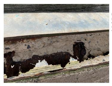
**Photo 2:** View on broken section of platform at edge support showing corroded Bondek sheeting and remnants of dovetail ribs embedded within the concrete
