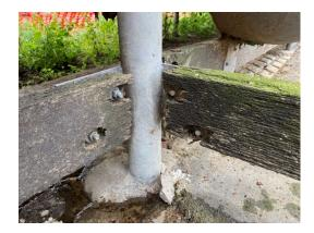
Material Decayed. Fixture Bolts Loose.
