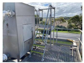
Photo 9: Large screen access platform and step-type ladder with handrail missing from one side of ladder and no barrier under platform protecting the exposed north edge.
