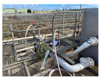
Photo 8: Small screen access platform and step-type ladder with non-compliant handrails, lack of toe-board to near side and mid-rail missing next to screen.
