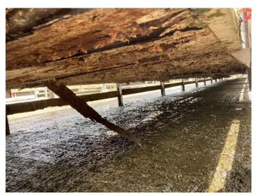
**Photo 4:** Different platform structure viewed from underside showing Bondek sheeting has corroded out and is collapsing away from the concrete.
