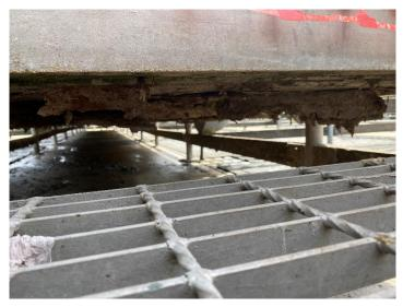
Photo 7: View under typical platform showing manure adhered to underside and Bondek sheeting starting to peel away from concrete.
