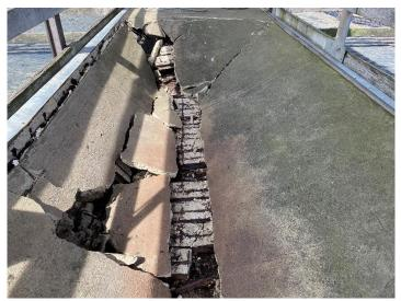
**Photo 1:** Collapsed section of platform.
