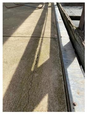
**Photo 5:** Longitudinal fracture line formed near support for platform where hogging moments are at their highest and failure of the platform is imminent.
