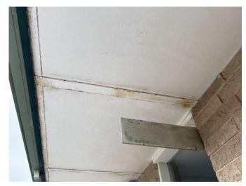
Photo 2: Minor surface corrosion to exposed Stramit beam.
