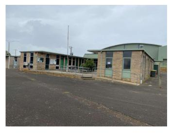
Photo 1: Administration building viewed from north west showing single story full masonry structure with flat pitched roof.
