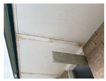
Photo 2: Minor surface corrosion to exposed Stramit beam.
