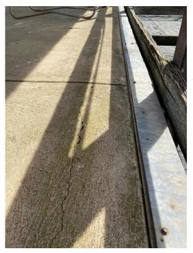
**Photo 5:** Longitudinal fracture line formed near support for platform where hogging moments are at their highest and failure of the platform is imminent.
