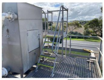
Photo 9: Large screen access platform and step-type ladder with handrail missing from one side of ladder and no barrier under platform protecting the exposed north edge.
