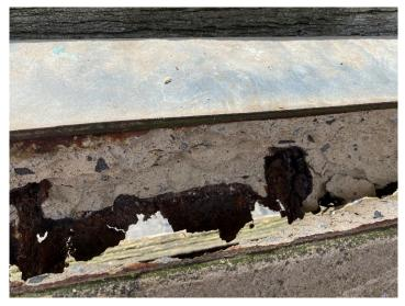
**Photo 2:** View on broken section of platform at edge support showing corroded Bondek sheeting and remnants of dovetail ribs embedded within the concrete
