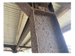
Facing E Portal column severely corroded.
