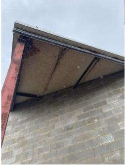
Photo 7: Corrosion of exposed column, purlins, bridging and soffit lining to dairy selling shed.
