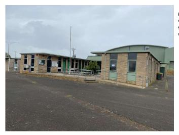
Photo 1: Administration building viewed from north west showing single story full masonry structure with flat pitched roof.
