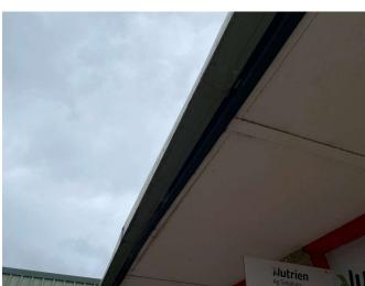
Photo 3: Dislodged guttering on west side of courtyard.
