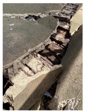
**Photo 3:** View on broken section of platform at midspan showing Bondek completely corroded through leading to brittle failure of concrete.
