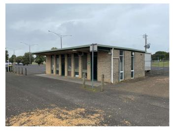
Photo 4: Store building (former bar) viewed from north west showing masonry external walls and a flat pitched roof.
