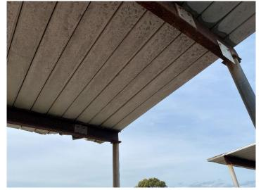
**Photo 6:** View of typical roof structure showing corroded support purlins and roof sheeting in single span arrangement over excessive distance for capability of sheeting.
