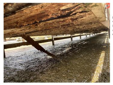
**Photo 4:** Different platform structure viewed from underside showing Bondek sheeting has corroded out and is collapsing away from the concrete.
