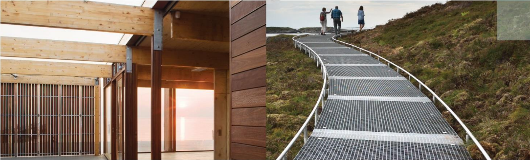
Hardwood timber - plantation - grown and recycled timber treated for protection from insects and decay - Red Gum, Jarrah and Tallowood are most durable and suitable for structure is the water. Photo: John Gollings Reinforced polymer mesh - lightweight - chosen for its excellent anti-corrosive and low maintenance properties. Photo: Roger Ellingsen
