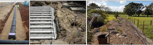
**Figures - 7-9** – ETA beds can be used with septic tanks to reduce and concentrate affluent disposal area; another useful upgrade option for small lots and aging systems (Source: Hydroscape 2019, William Cromer 2019, Mornington Peninsula Shire Council 2015).
