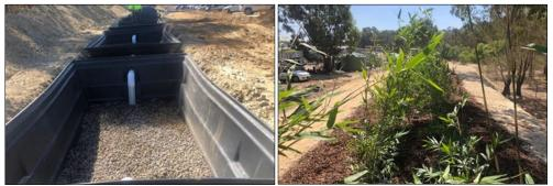
FIGURES 15-16 - Potential disposal solution (Rhizopod containment system) within constrained sites.
