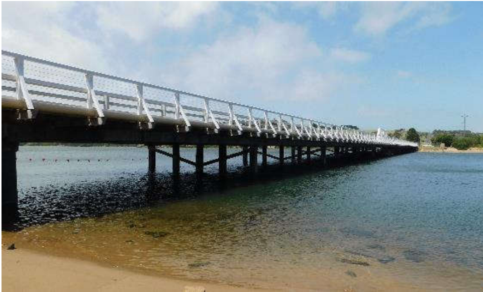
Figure 14: New Hopkins River Bridge – replicated timber railing and pier bracing (taken November 2020)
