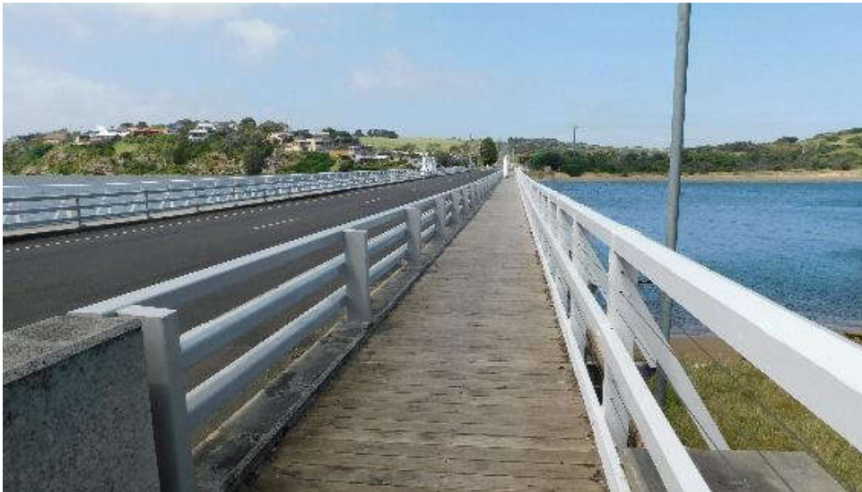
Figure 15: New Hopkins River Bridge – timber footpath railing (taken November 2020)
