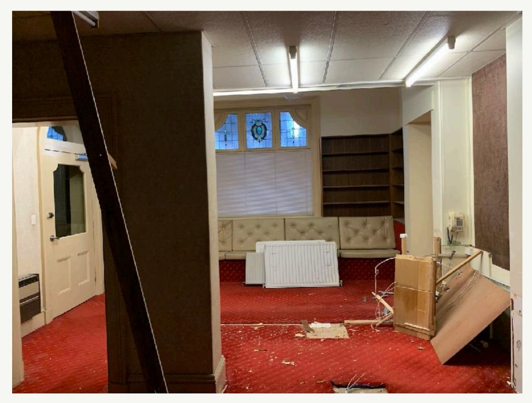
Existing first floor - infill ceiling to be removed and original ceiling heights restored, re-finish floor and fit out for Document Set ID: 11107389 Seating area
