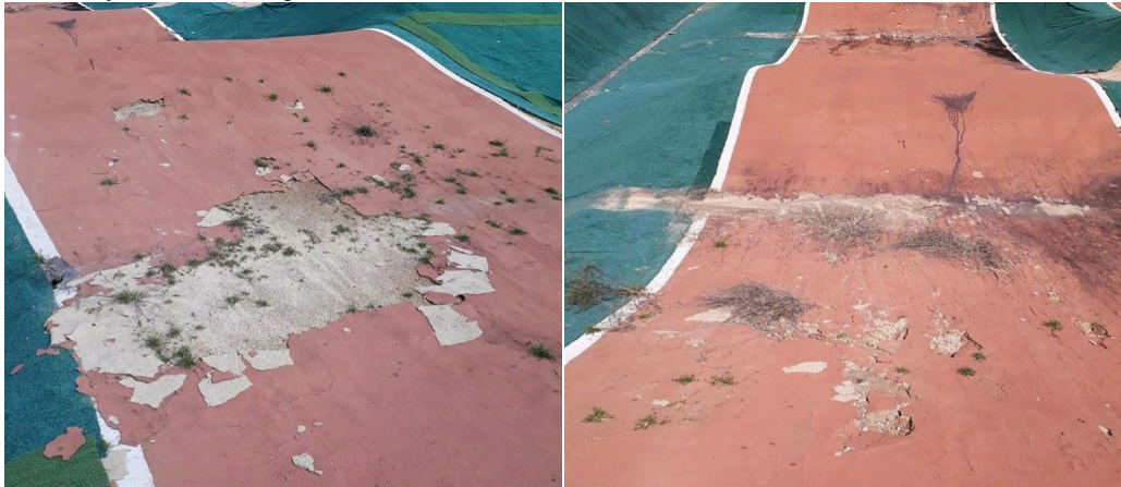
Photo: Soil stabiliser peeling off on BMX track leaving the original granitic sand exposed.
