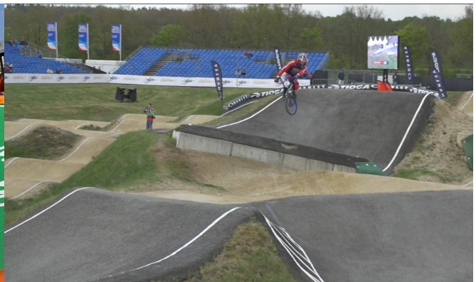
Photo: (Left) the section of this BMX track has been concreted and painted green. Photo (Right) the sections of this BMX track have had bitumen applied to them.
