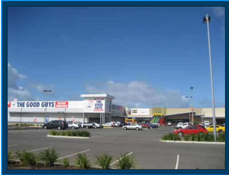
PHOTOGRAPH 3: THE HOMEMAKER CENTRE: STREET-FRONTAGE
