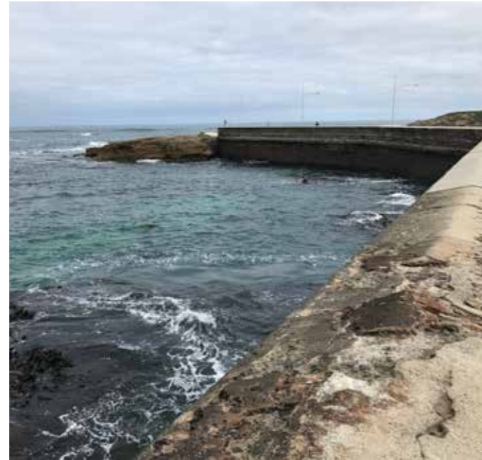
The breakwater is a historically significant part of the coastline. Existing facilities are degraded and regular maintenance and capital works is required to maintain its structural integrity.
