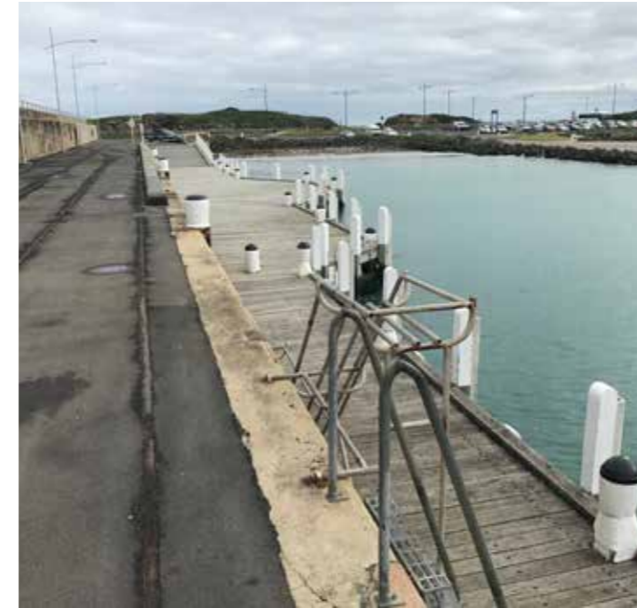
Modifications to boat launch area needs to consider the function and use of existing platforms and historic significance of the breakwater.
