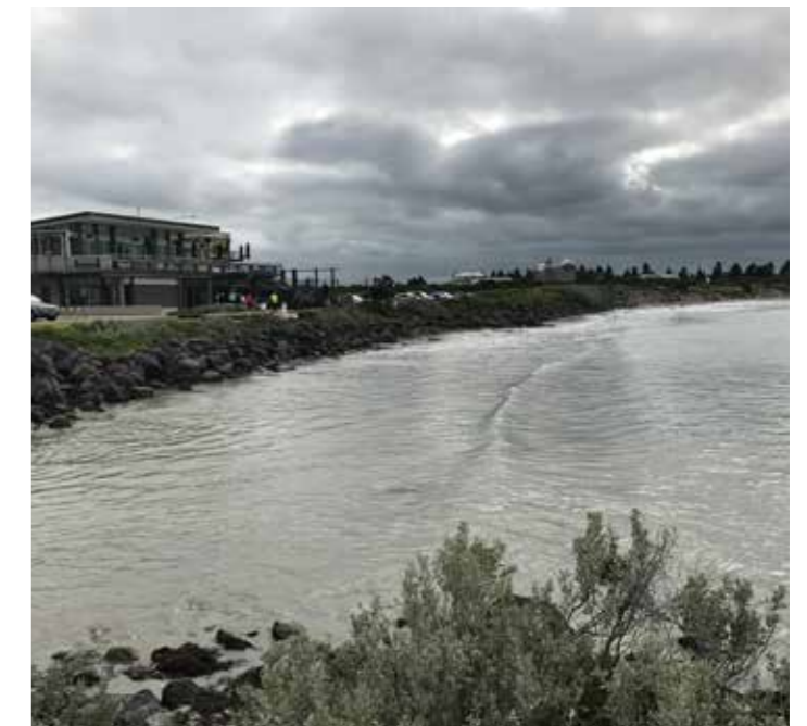
Rock work provides protection from coastal processes but also creates a buffer between pedestrian areas and the beach.
