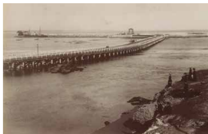
The breakwater, c.1892-1902. Source: State Library of Victoria
