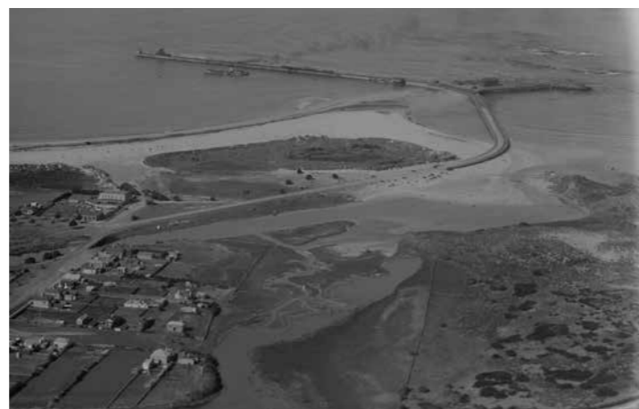
The breakwater, c.1925-30. Source: State Library of Victoria
