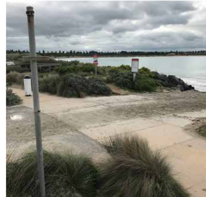
Northern boat ramp relatively steep and experiences regular erosion at the base. Sand dispersal has an impact on trail users.
