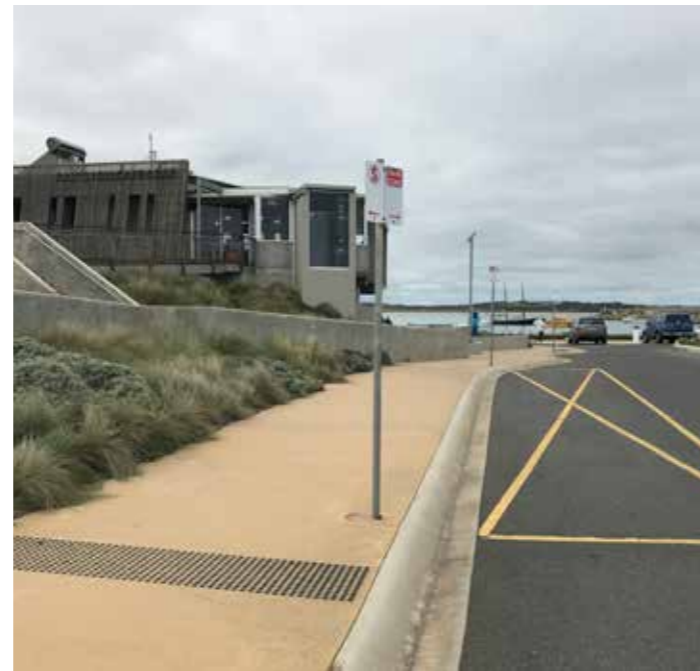
Bus parking has direct connection to pedestrian paths.
