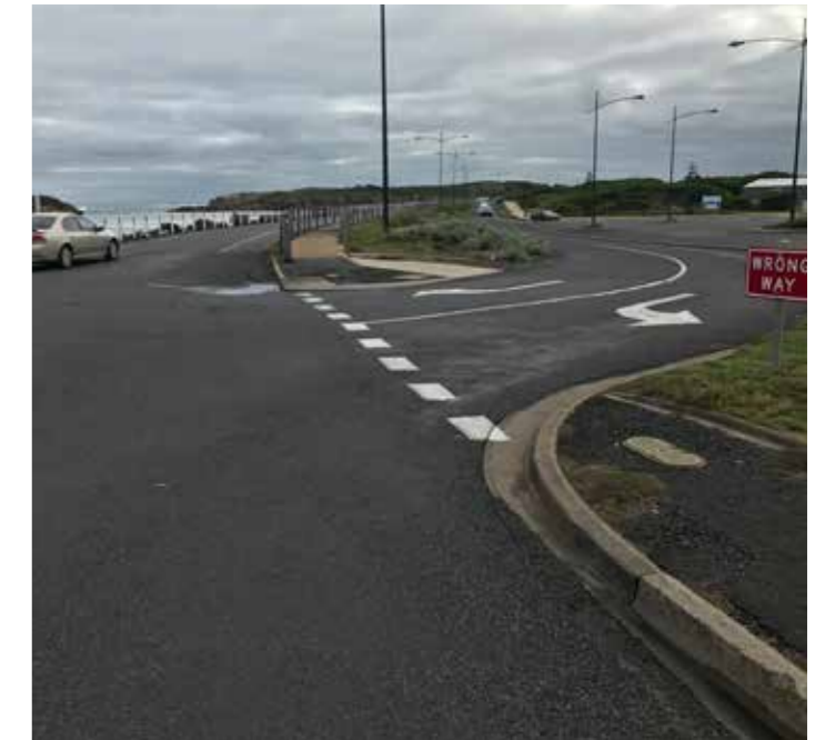
Confusing road network makes identification of car park circulation and exits difficult for visitors to the area.
