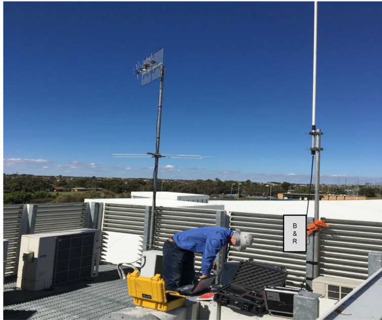
Figure 25. TFFWS base station testing on Aquazone Roof November 2016 (BoM, 2016)
