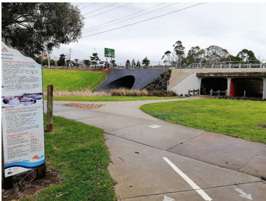
Figure 12. New high flow culverts to right of image 19 July 2018
