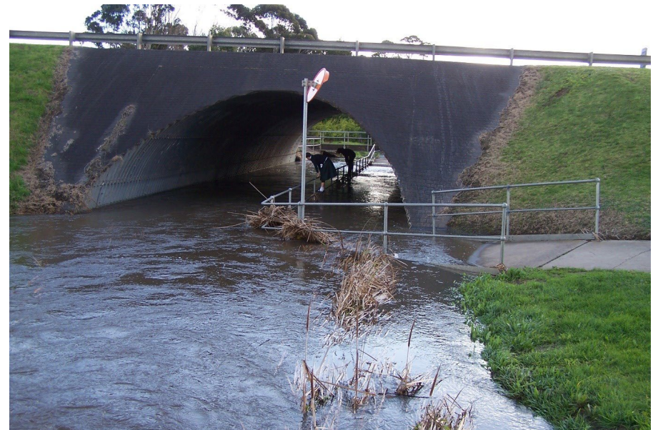
Figure 11. Russells Creek Mortlake Road original culvert 12 August 2010 3
