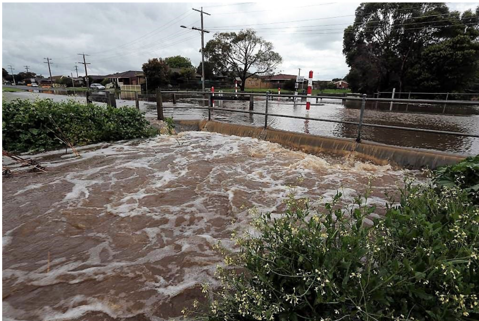
Figure 41. Queens Road crossing in flood 1
