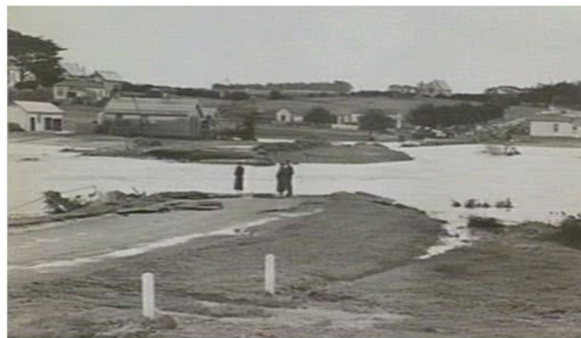
Figure 6. Woodford bridge washed away March 1946
