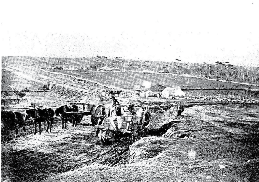
Figure 3. Road making Mortlake Road circa 18662 (Russells Creek in background).
