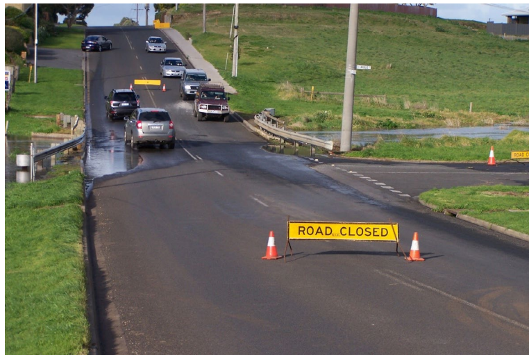
Figure 10. Daltons Road bridge 12 August 2010 3
