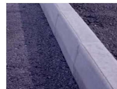
Charcoal coloured pigment concrete to match the bluestone kerbs. Use in highway streets and new/upgrade works to residential streets and carparks.
