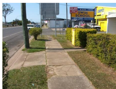
Condition 5 "Very Poor"
