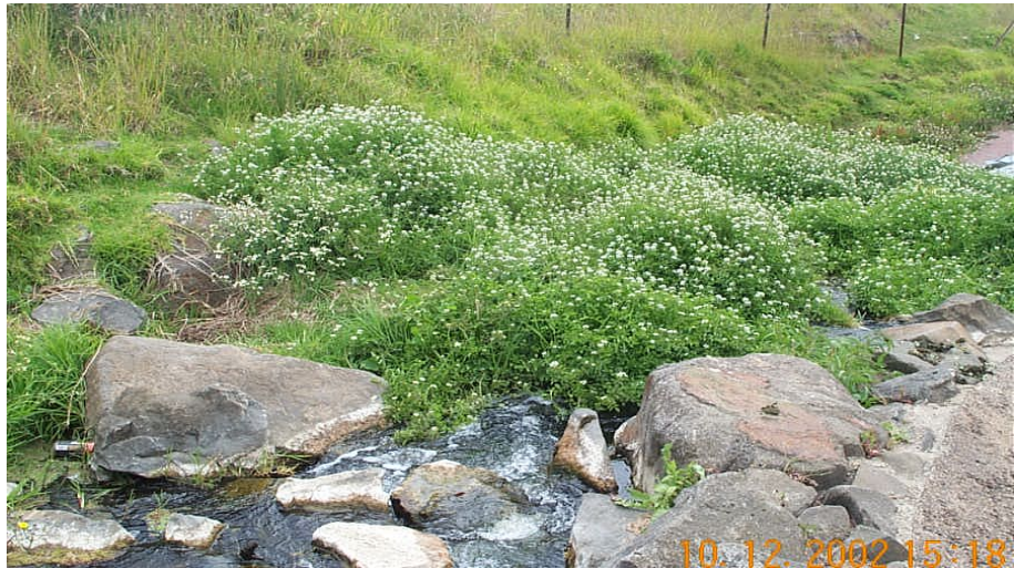
PHOTO 10: FISH LADDER & WEEDS AT THE WEIR.
