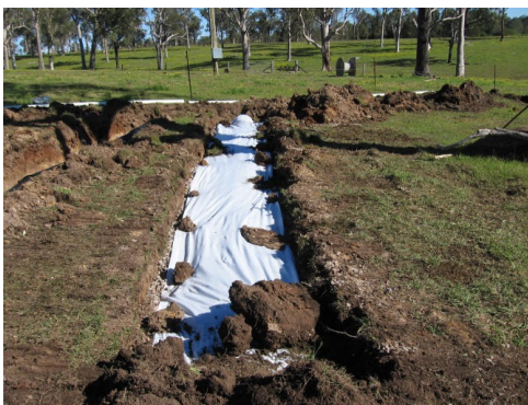
Figures 19 & 20: Latter stages of installation of soil absorption trenches (Source: Civcon 2019); soil mound effluent disposal (SCA 2019).
