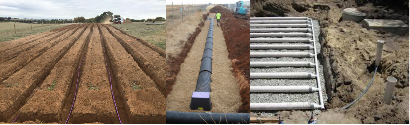
Figures 16-18: ETA beds can be used with septic tanks to reduce and concentrate effluent disposal area; another useful upgrade option for small lots and aging systems (Source: Hydroscape 2019, William Cromer 2019, Mornington Peninsula Shire Council 2015).
