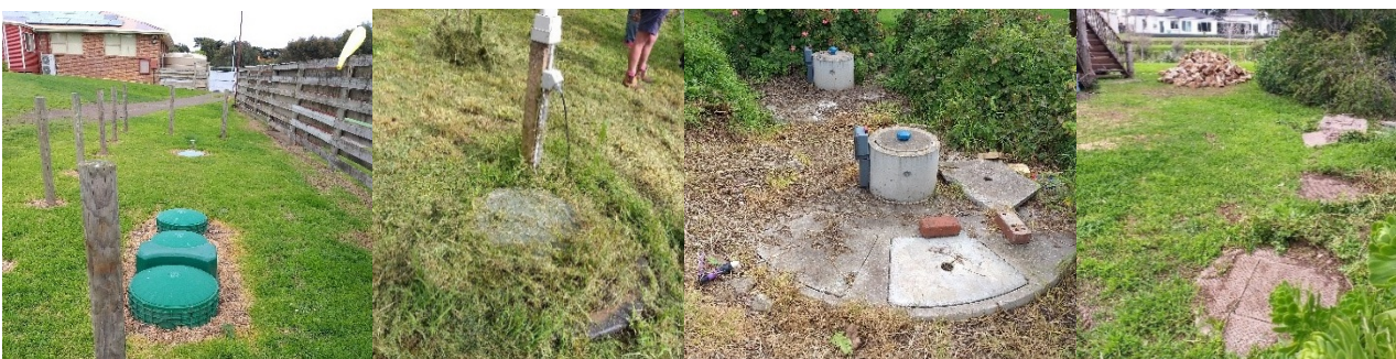
Figures 39-42 – Systems within watercourse setbacks evidenced during DWMP audit; all locatable, managed, and maintained therefore reducing operational risk.
