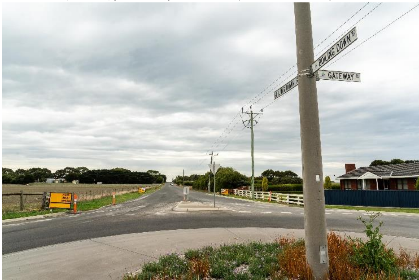
Boiling Down Road was reconstructed in early 2019.
