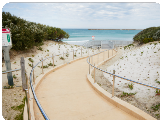
Another access within the McGennan Car Park area, Beach Access 122, saw some timber renewal.
