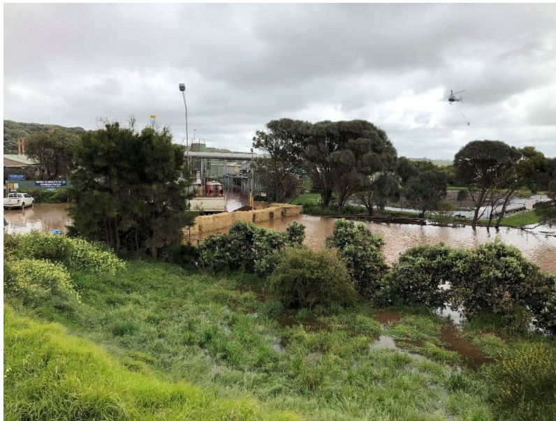
Figure 1-12 Photo of flooding temporary levee at the Midfield Meats Rendering Plant with helicopter dropping sandbag
