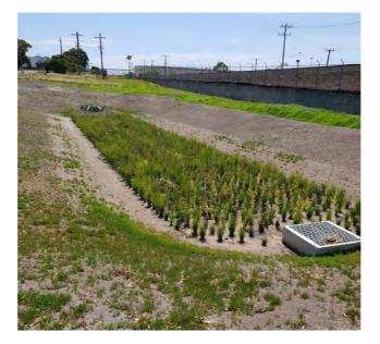
Figure 18: Bio-basin at base of retardation basin
