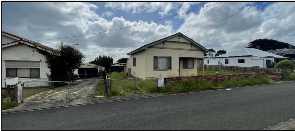
Image 2: View of subject site from Preston Street – looking north west.
