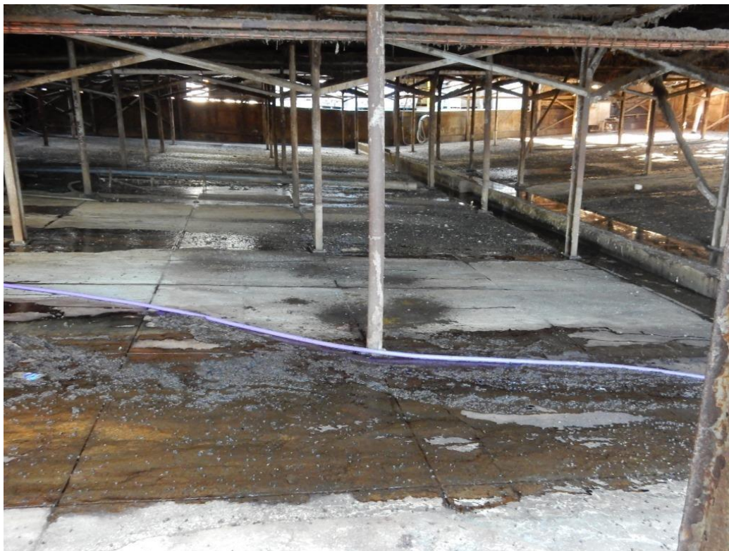
Sheep lairage showing condition of floor under grills, with sloping floors for drainage.
