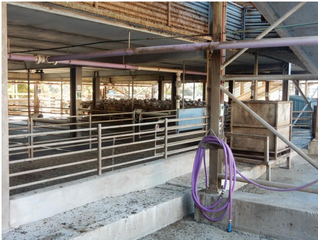
Sheep lairage showing condition of floors and cleaning provisions (purple hoses and lines)
