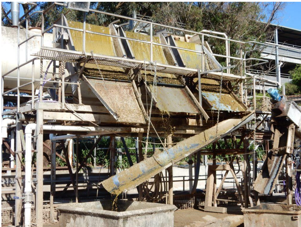
Existing screens (green/paunch line), wastewater treatment plant.
