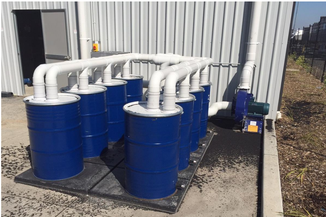
Figure 12: Example of carbon filter drum unit installation. Only two such units will be required to treat air extracted from the DAF headspace.
