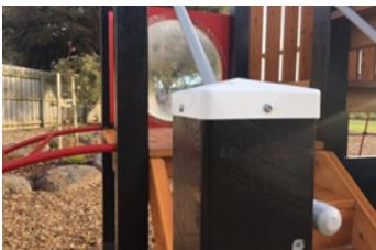
All timber posts will be fitted with a PVC cap that should prevent moisture penetration.
