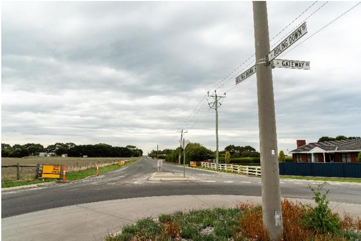
Boiling Down Road was reconstructed in early 2019.
