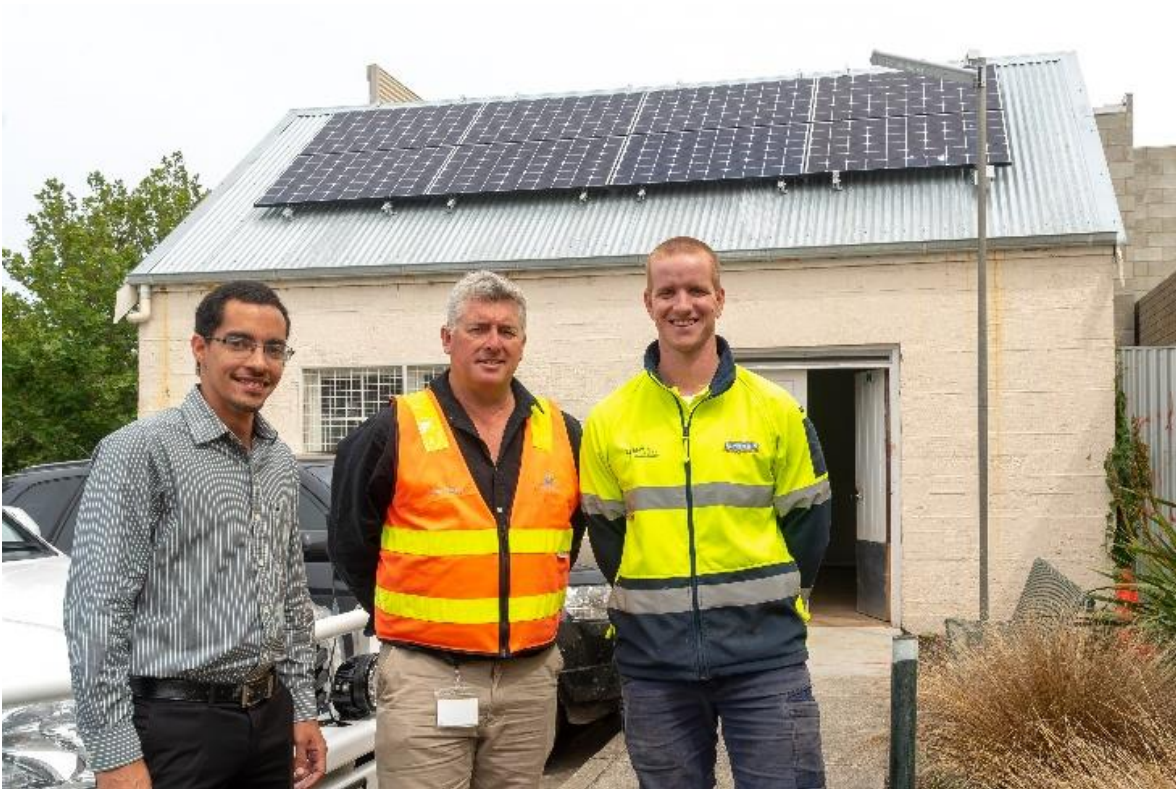
The off-grid solar installation in Ozone Car Park.
